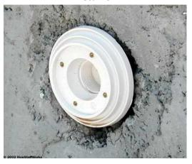
How it Works: returns filtered water to pool from the pump
